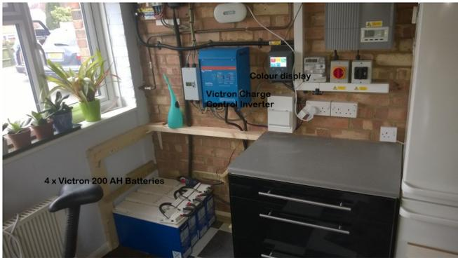
The Batteries, although being relatively heavy, are compact and more capacity can be easily added. The system does not change the FIT payments in any way because the PV energy has already passed through the generation meter before going to the batteries (unlike the DC Charge Inverter systems such as Growatt or Tesla)
